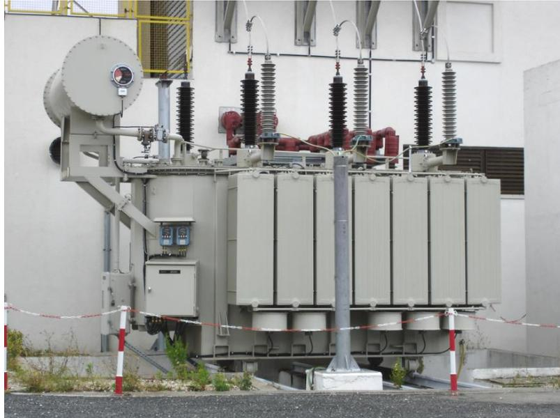
Slika 2. 6: Transformator 110/10 kV, 68,5 tona, 15 tona ulja
